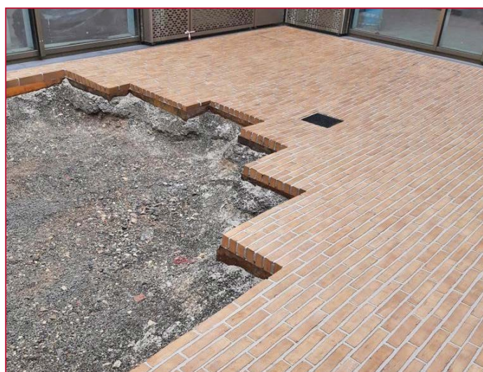
Immediately after sweeping, a clear joint pattern is visible
