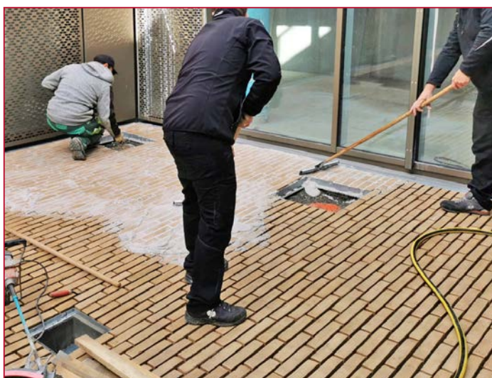
Processing of the joint mortar according to the instructions of the ROMEX® technician on site
