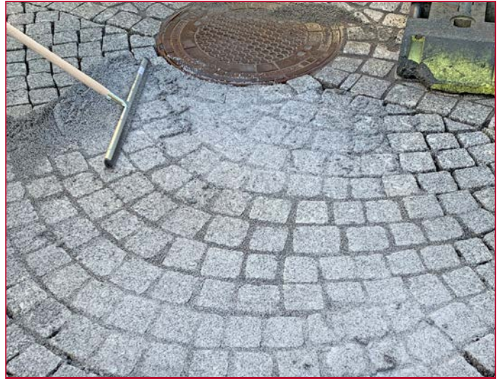
Jointing with ISATEC® - FLEX, colour stone grey
