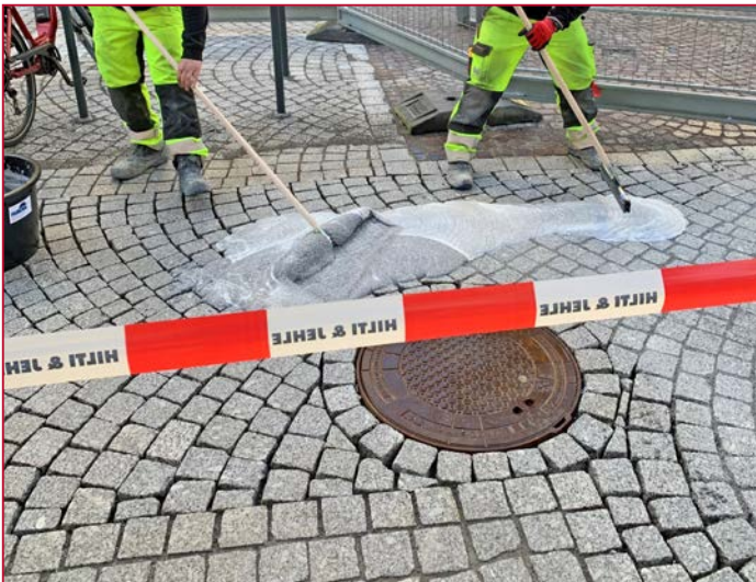
Efficient jointing in teams of two
