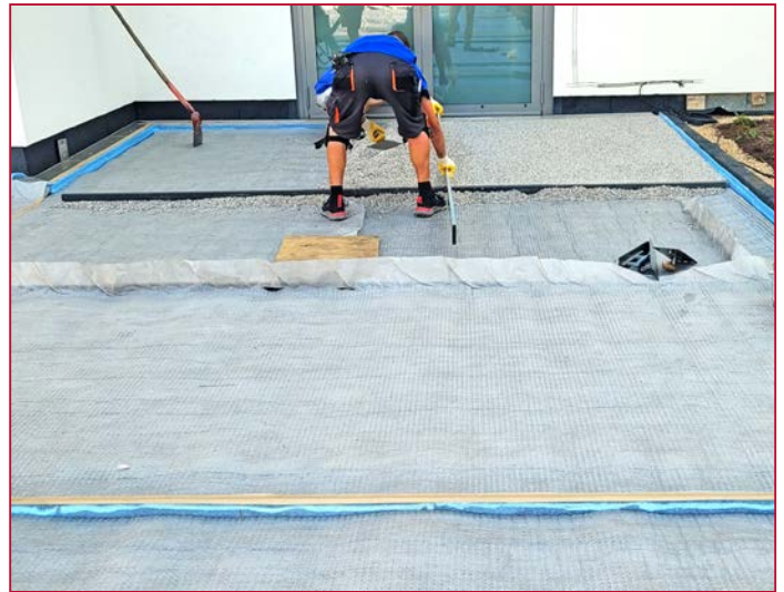
Geotextile as a separating layer under the gravel
