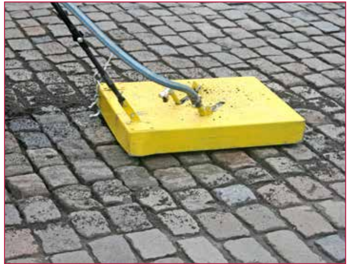
Fugen reinigen | Clean the joints
