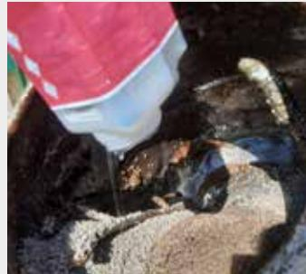
The products ROMPOX®- 201 DEKO UV and ROMPOX®- 202 DEKO EP were then used to professionally apply longitudinal strips to all superstructures. The product ROMPOX®- 201 DEKO UV was applied with two white marble grits a) 4/7 mm and b) 2/4 mm with 5% binder content each, ROMPOX®- 202 DEKO EP with brown granite grit 3/5 mm and 6% binder content.
